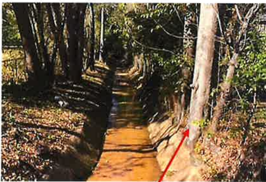
Buffer Area Encroachments
