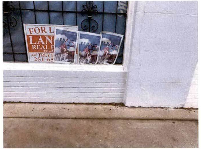
14. detail view of area of non-original bulkhead at western-most subject property
