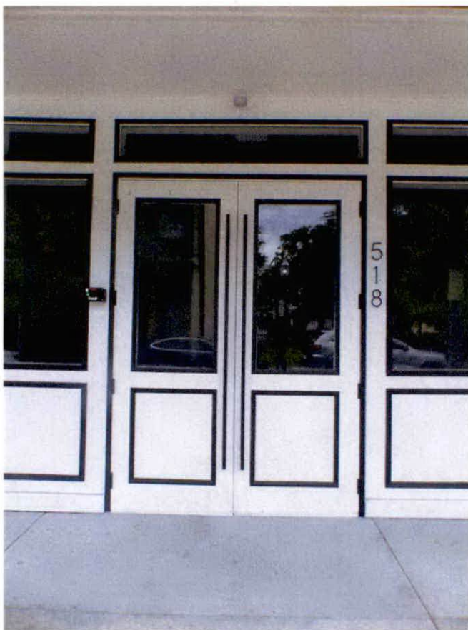
9. view north to doors installed as proposed at 518 (formerly 508) Dauphin Street (6/7/2022)
