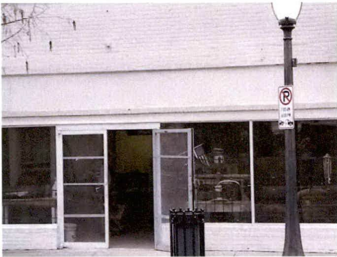
13. detail view of storefront in eastern subject property
