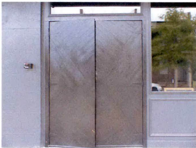
7. detail: installed doors on south elevation of 518 Dauphin Street (6/7/2022)
