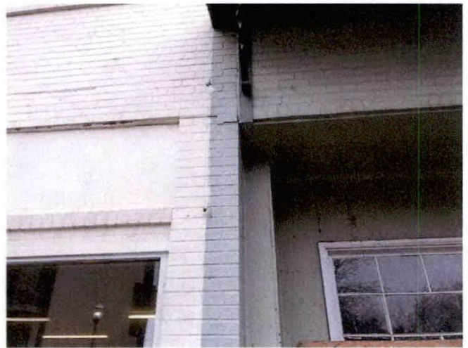
10. view north to junction between easternmost subject property and adjacent unit (note no apparent transom at right)
