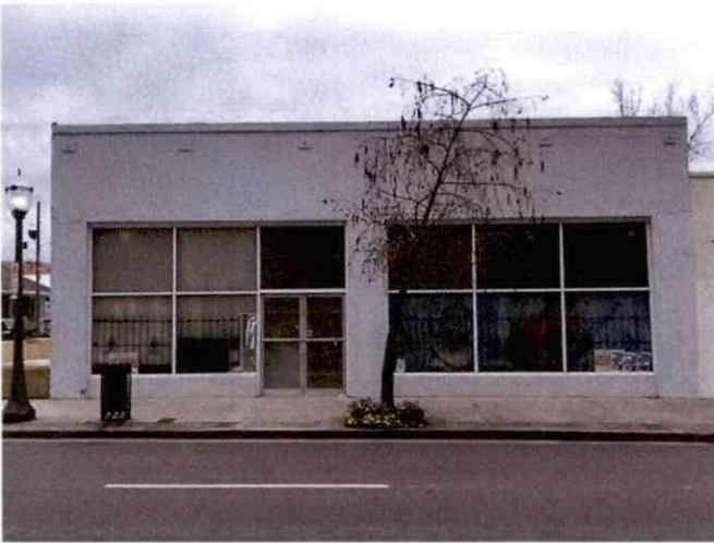
1. south elevation of westernmost building (2/2021)
