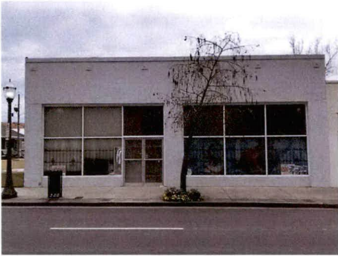
1. south elevation of westernmost building
