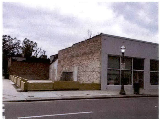
4. view north-northeast to west elevation of subject property
