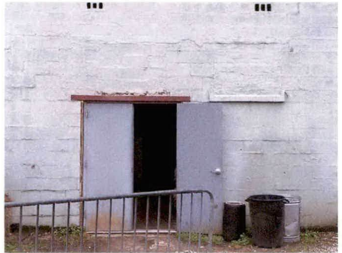
8. detail view of area of proposed fenestration change on rear (north) elevation
