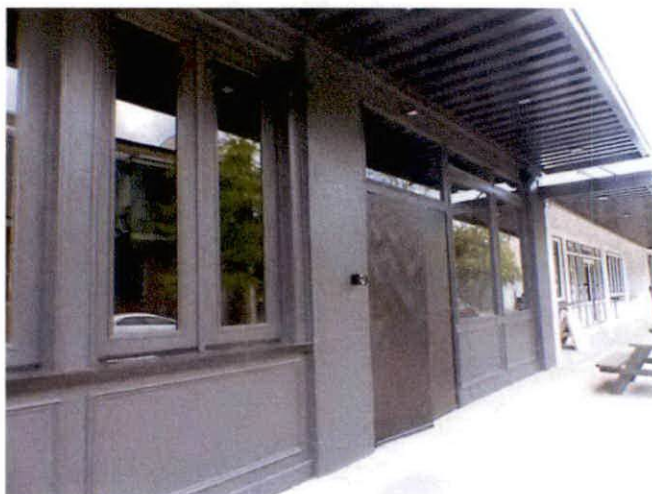
8. view northeast to south elevation (façade) of 518 Dauphin Street; 508 Dauphin at right (6/7/2022)
