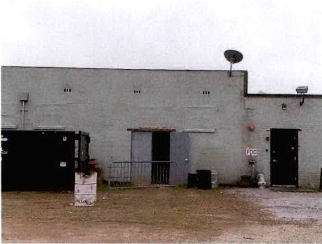
7. view south to area of proposed fenestration changes on the north elevation of the subject property
