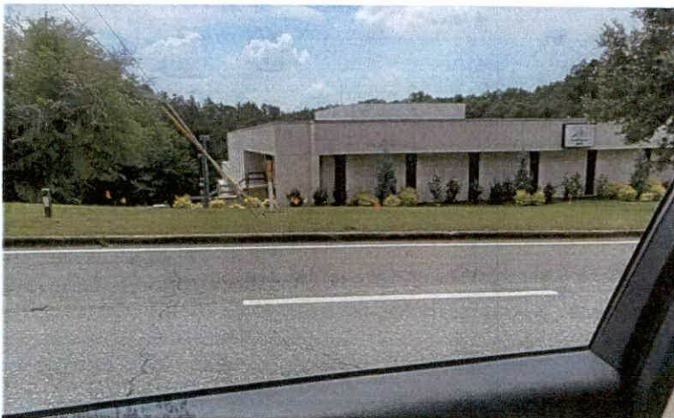
1016 Hillcrest Rd B-3 multi Office building
