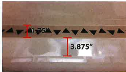
Image #17 - The support brace on the top shelf is 1 \frac{3}{4} " high and is 3 \frac{7}{8} " deep
