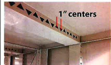
Image #18 - The support brace is 36" wide and has triangle shapes at 1" centers
