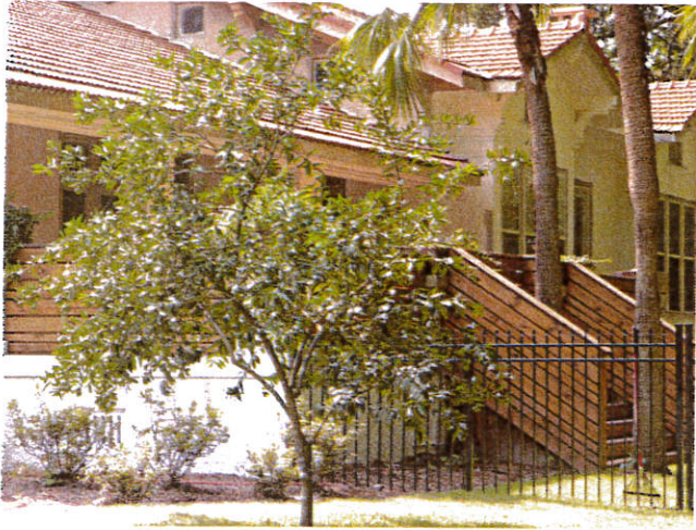
6. East Elevation, Northwest View as of 7/26/2018
