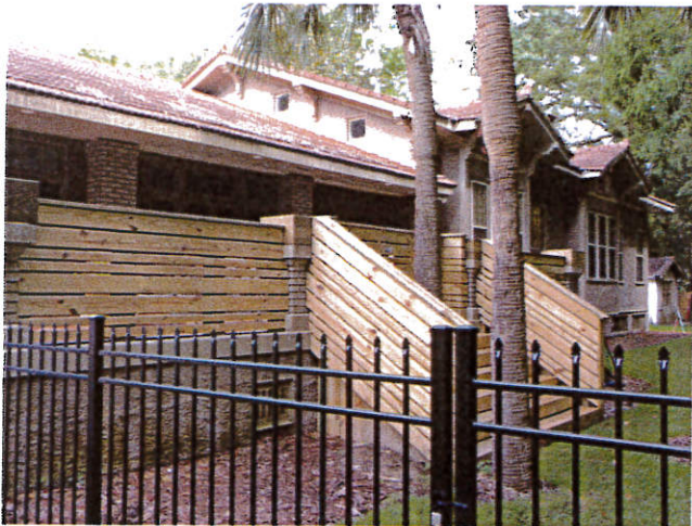
3. East Elevation, Northwest View
