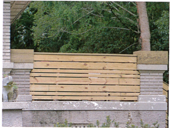
2. Close up of railing on South Elevation
