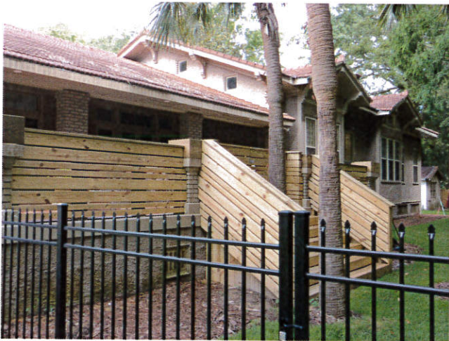
3. East Elevation, Northwest View
