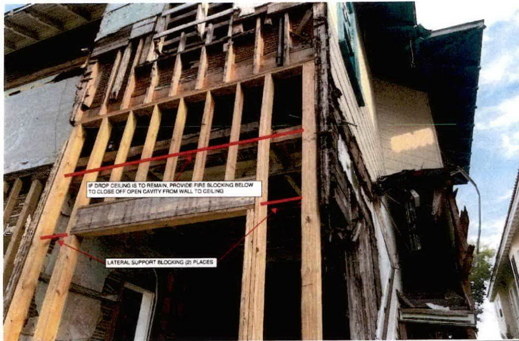
Figure 1. Blocking for South-East Wall
