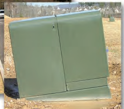
Leveling Pad-Mounted Equipment
