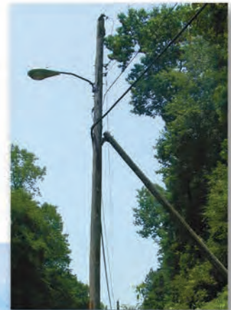
Push-Brace Support Poles
