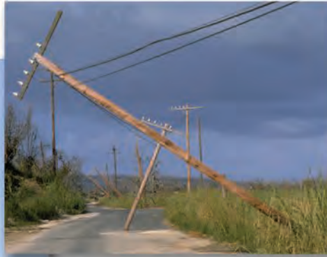
Repairing Storm Damaged Poles
