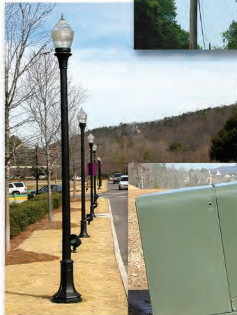
Installing or Straightening Decorative Street Lighting
