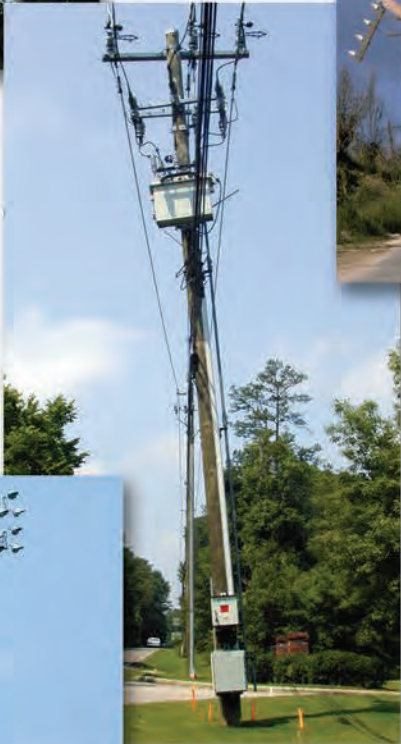
Straighten Leaning Poles
