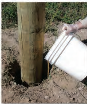
Pour mixture in prepared hole with pole.
