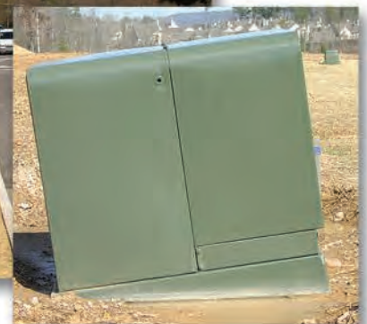
Leveling Pad-Mounted Equipment
