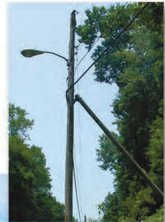
Push-Brace Support Poles
